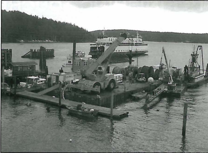
Caldwell Marine International's barge was trucked to the West Coast in pieces and put together at the Port of Tacoma. It was then transferred by water to Orcas Landing.
